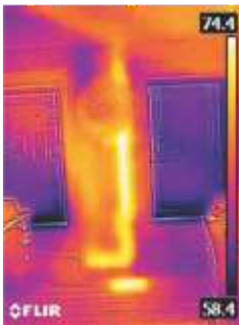
Warm Drain Pipe in Wall
