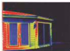
Infrared Thermograph for exterior building walls' heat leakage
